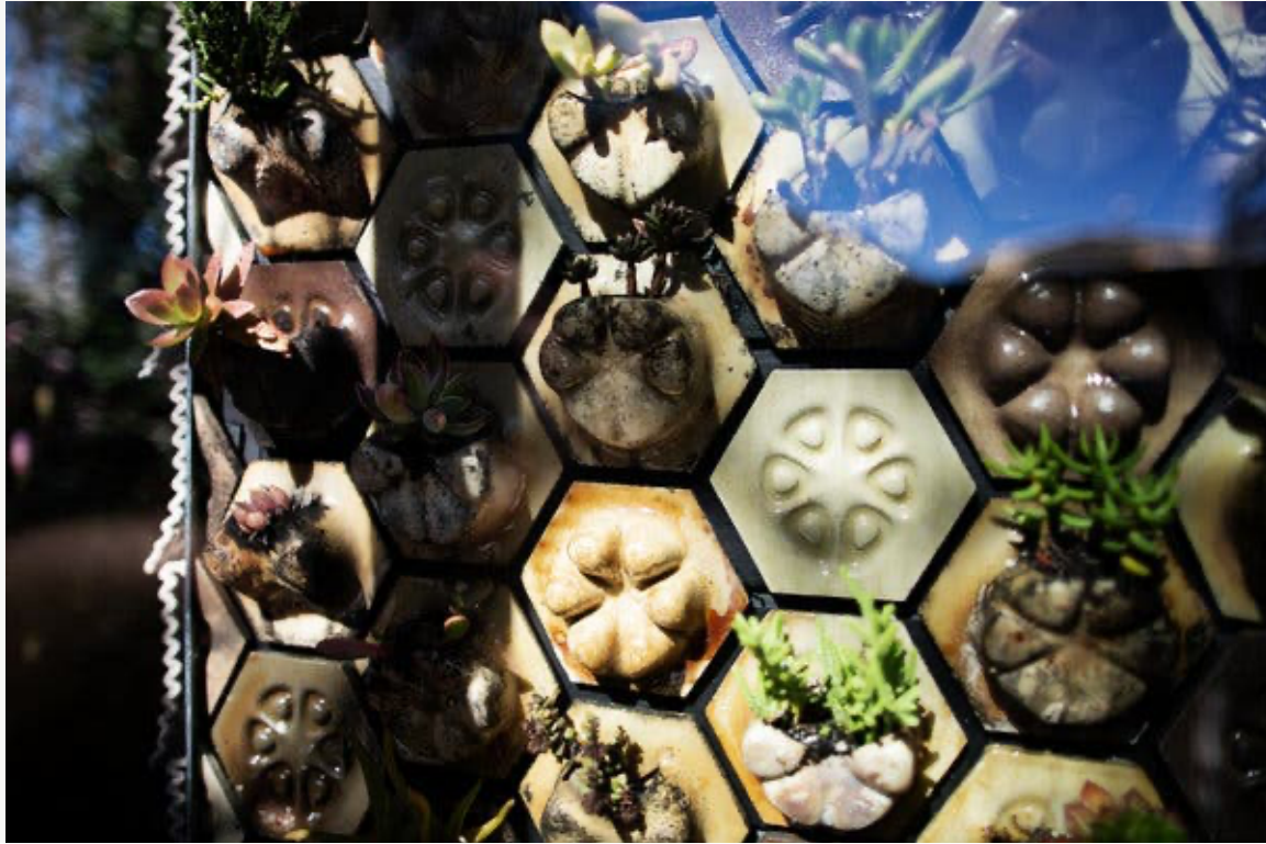
The cabin's 3-D-printed planter tiles (made of either chardonnay grape skins, sawdust or cement), with succulents along the front of the cabin. Credit... Talia Herman for The New York Times
